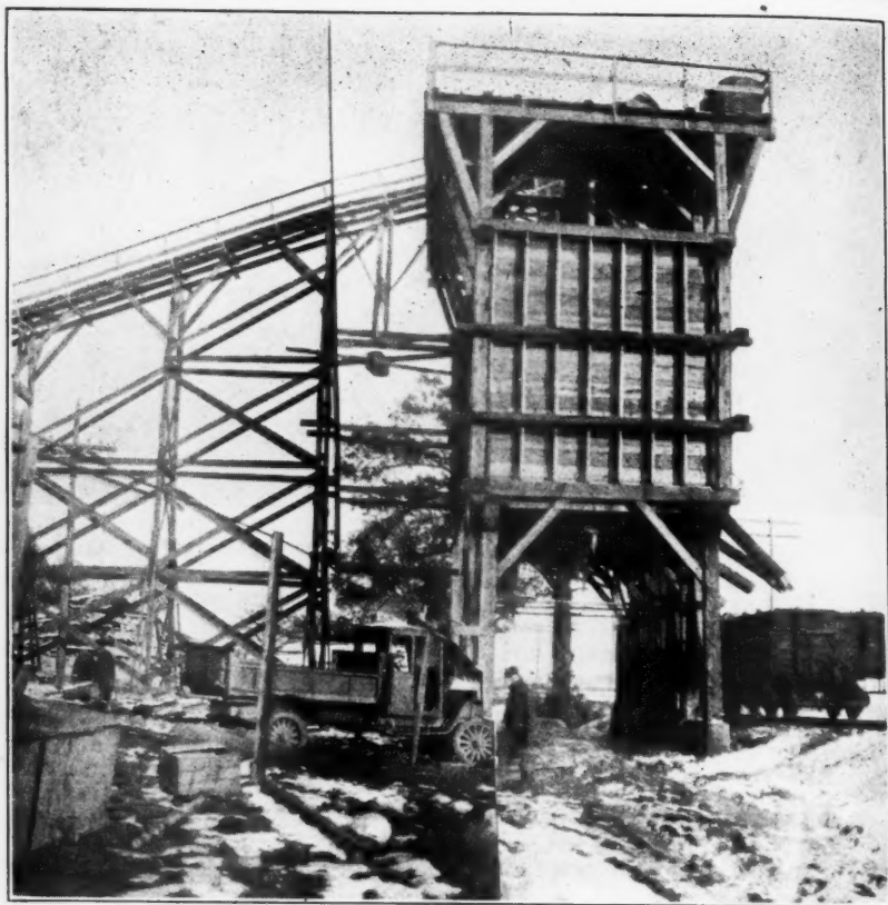
End View of Bunkers Showing Loading Facilities
